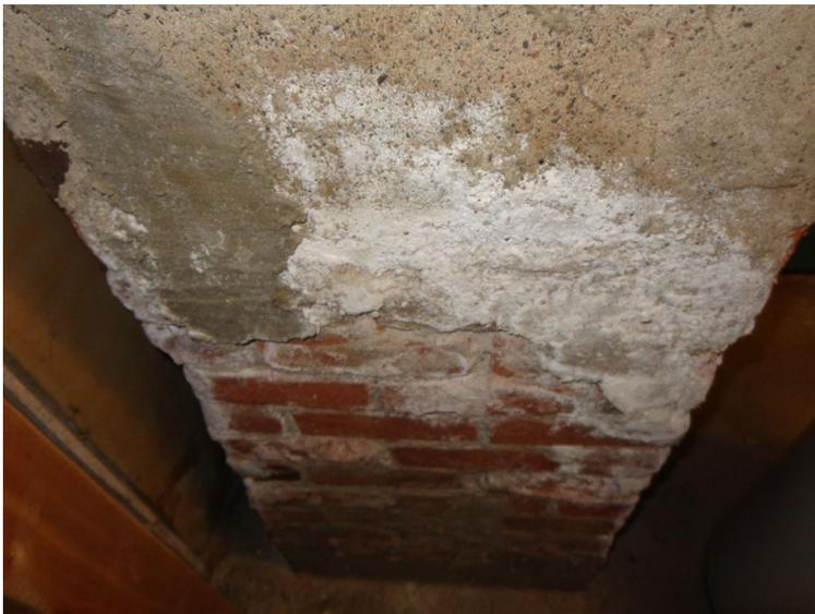
Photograph 7: View of the deteriorating chimney in the boiler area with efflorescence present, an indicator of elevated moisture content.
