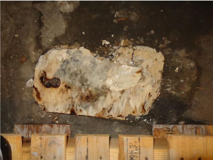
Photograph 3: View of deteriorating cardboard and water-stained wooden pallet on floor in northwest corner of the basement.
