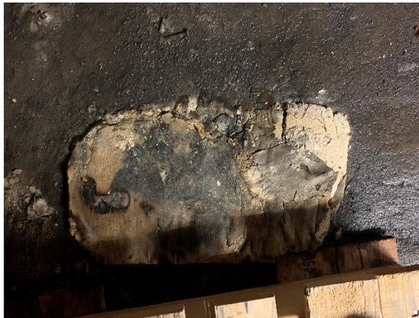
3. Extensive mineral efflorescence was found throughout the entire basement – the efflorescence clearly shows as a water line in the boiler room. The extent of the efflorescence indicates multiple water intrusion events.
